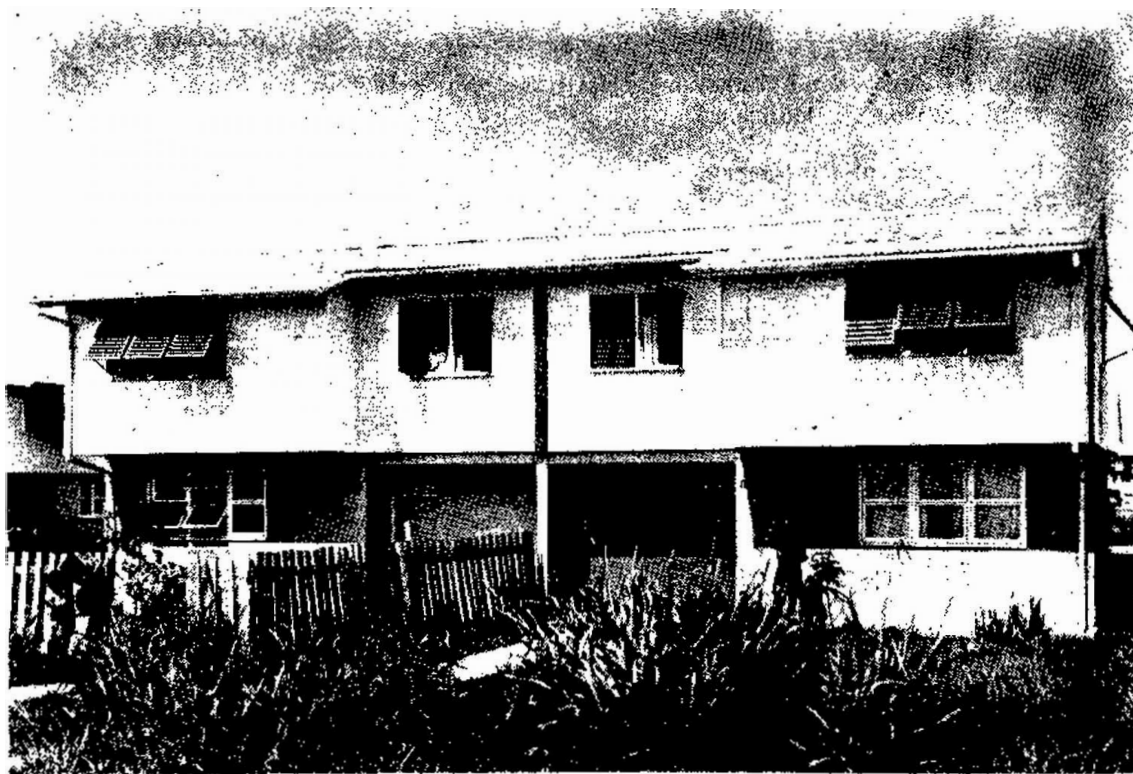
Duplex House at GUYHOC PARK, East La Penitence.
