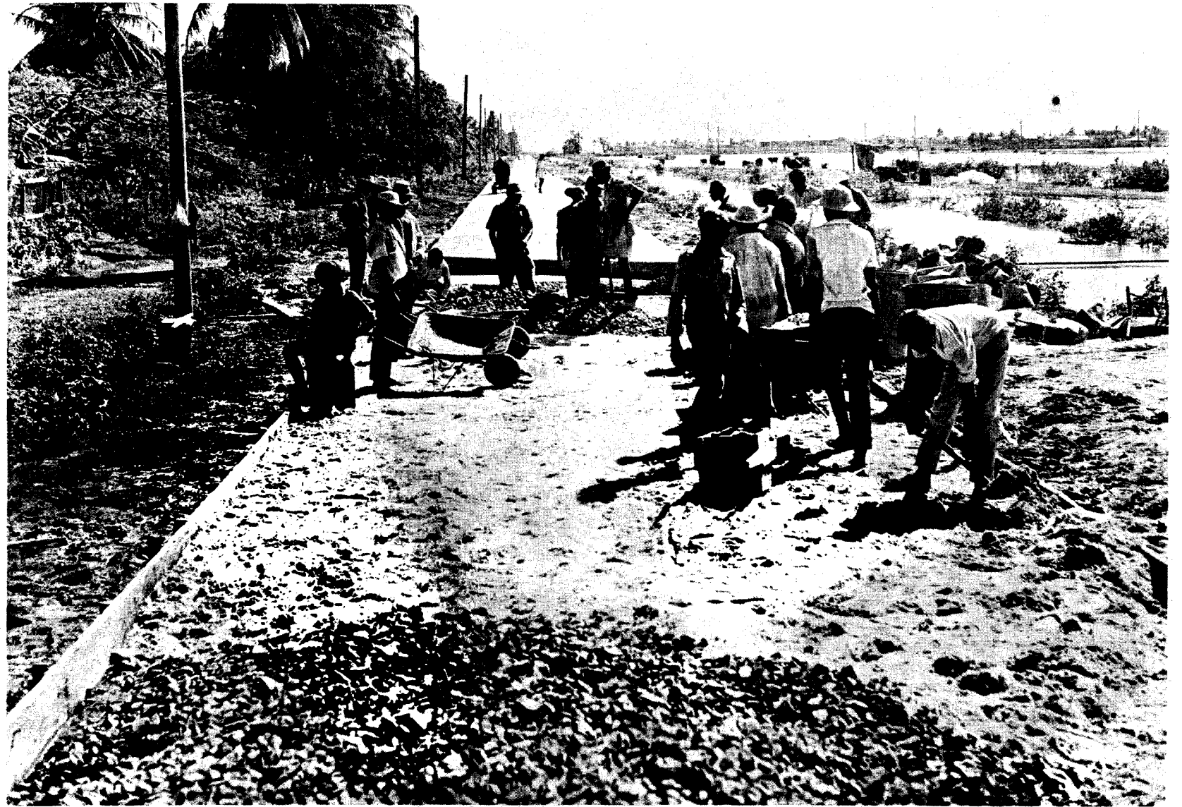
Construction of the Enterprise New Road, East Coast, Demerara in Progress
