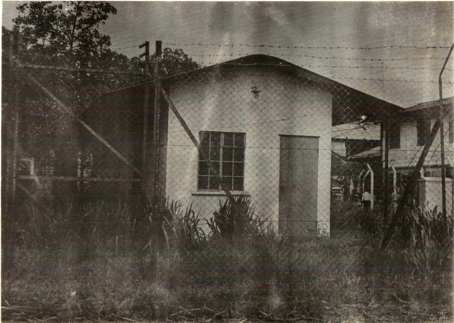
A Typical Unit Automatic Exchange (U.A.X.) Building.
