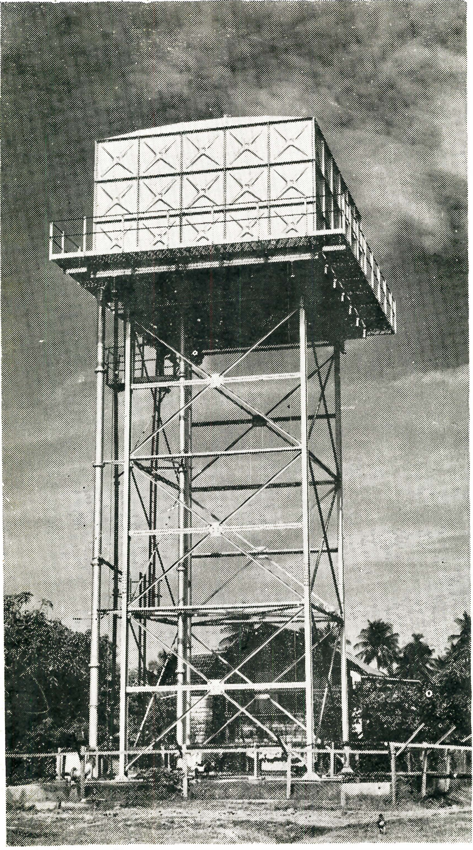
Overhead water storage tank at Enterprise, Non Pareil Estate.
