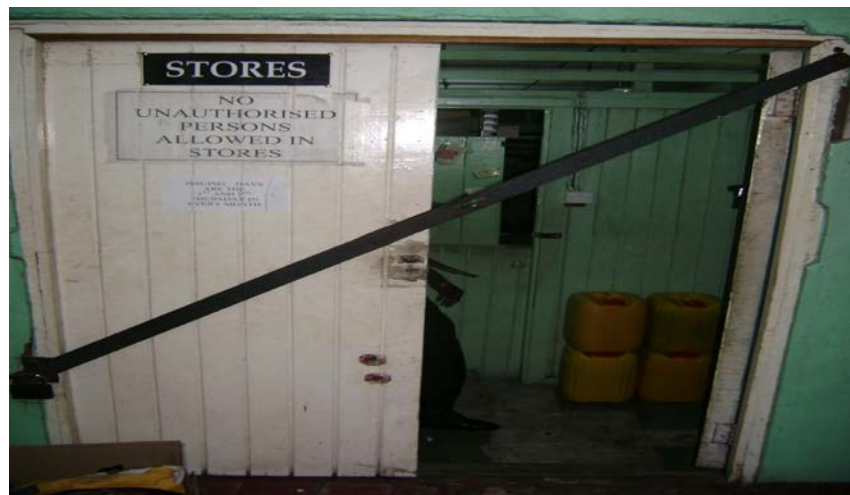
Fig. 5 – MLHSSS Entrance to Stores (Photographed 29/09/09)
