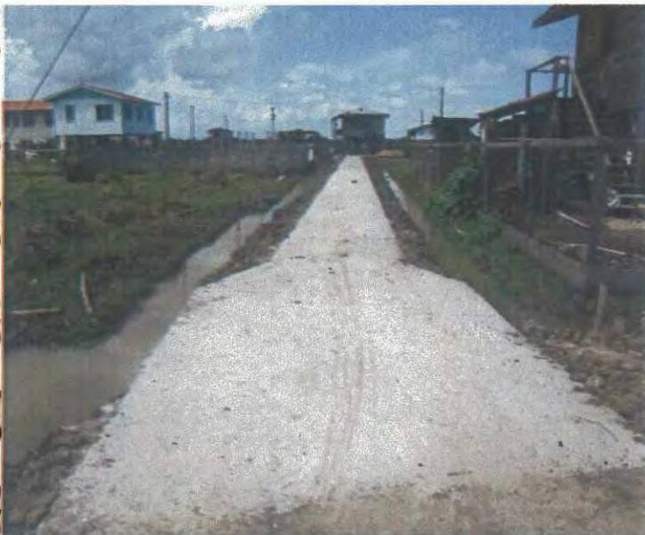
Completion of Walk-way
