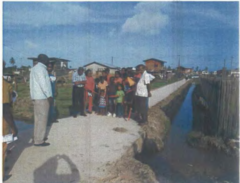
Opening of the Concrete Walkway
