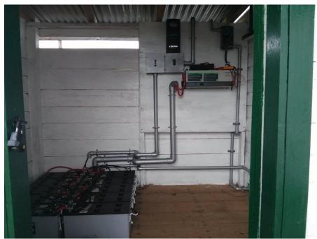
Picture showing completed installation of the Stand-alone PV system for the health centre
