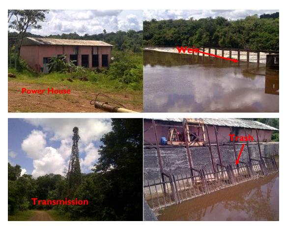
Components of the Hydropower Plant
