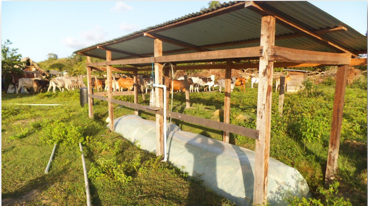
Biodigester Constructed at Rupertee
