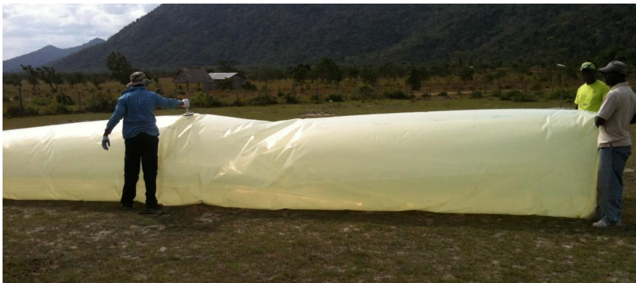
Assembling the biodigester plastic
