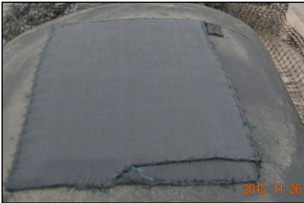
Figure 1: Section of repairs completed on Victoria Geo-tube breakwater
