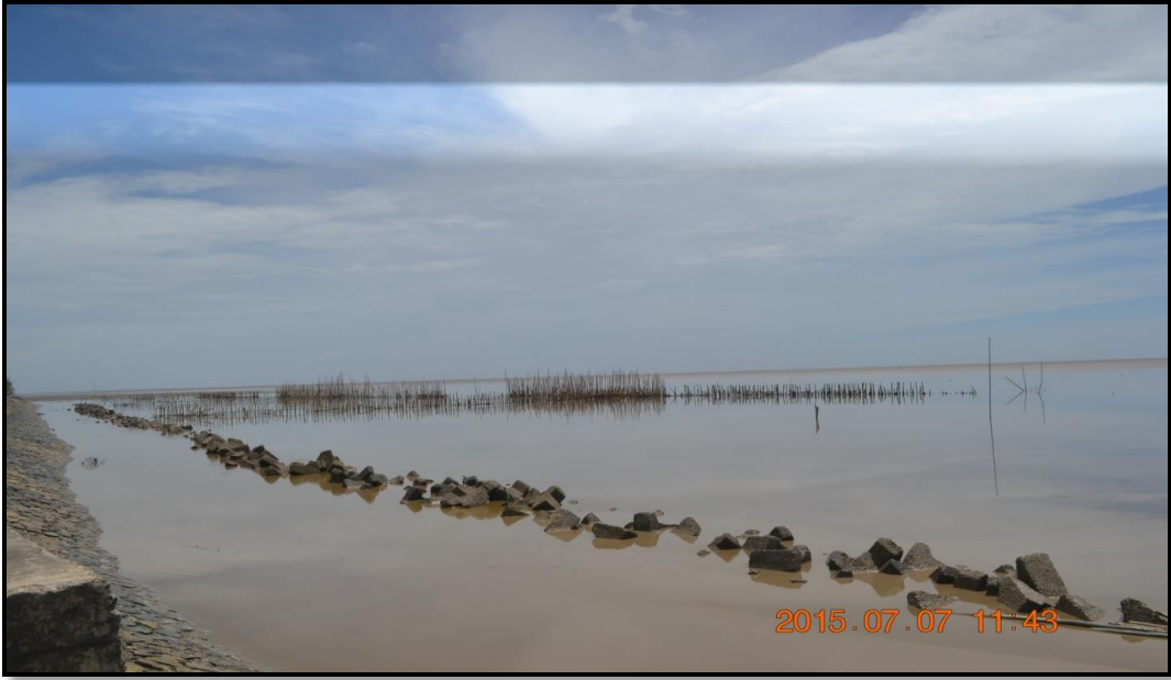
Figure : Repairs completed to Buxton Bamboo Brushwood Dam
