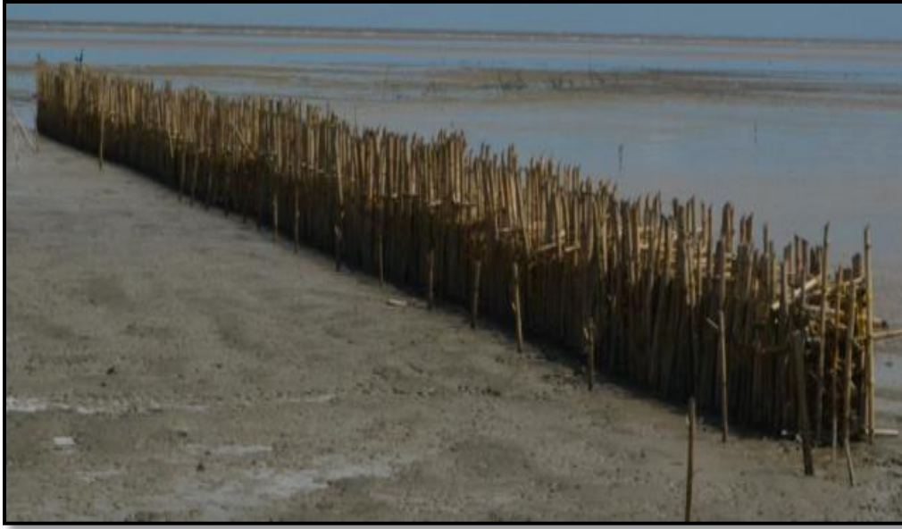
Figure: Completed Walton Hall Bamboo Brushwood groyne
