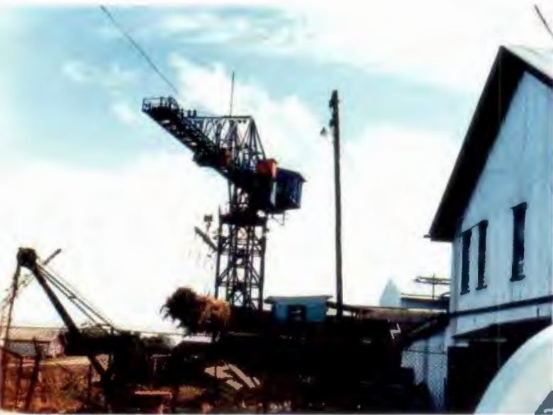
A typical factory facility
