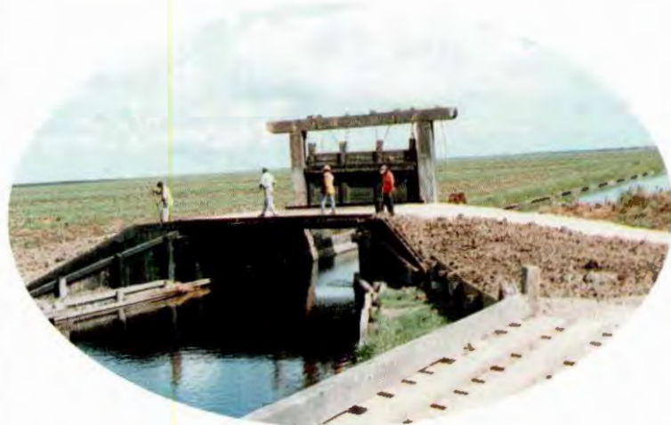
Costly infrastructure provides access to the No. 43 Koker Expansion Project.
