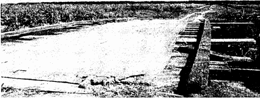
Figure 1 Showing VB'N 28 High Bridge – Deck had to be covered utilizing old punt bottom
