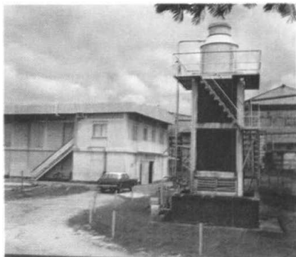
The Vinegar Plant Building
