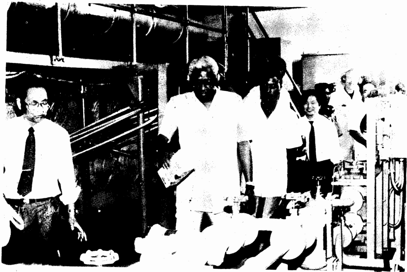
G.E.C. 5.8 MEGAWATT GENERATOR AT GARDEN OF EDEN
