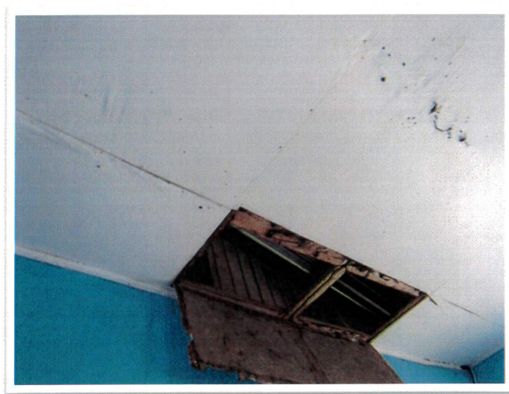
Figure 10 - Picture showing dilapidated ceiling at Agatash Primary School
