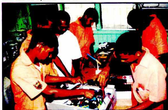
Apprentices of the Instrumentation Section of the GuySuCo Training Centre work on UPS's under the supervision of an instructor.
