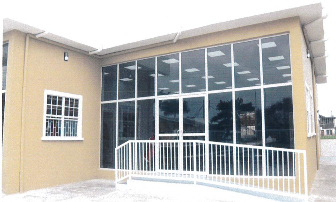
Figure 3- The Sophia Care Centre's kitchen upgraded in 2022.
